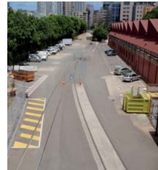
View from pedestrian overpass
