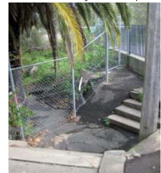
Access to light rail
